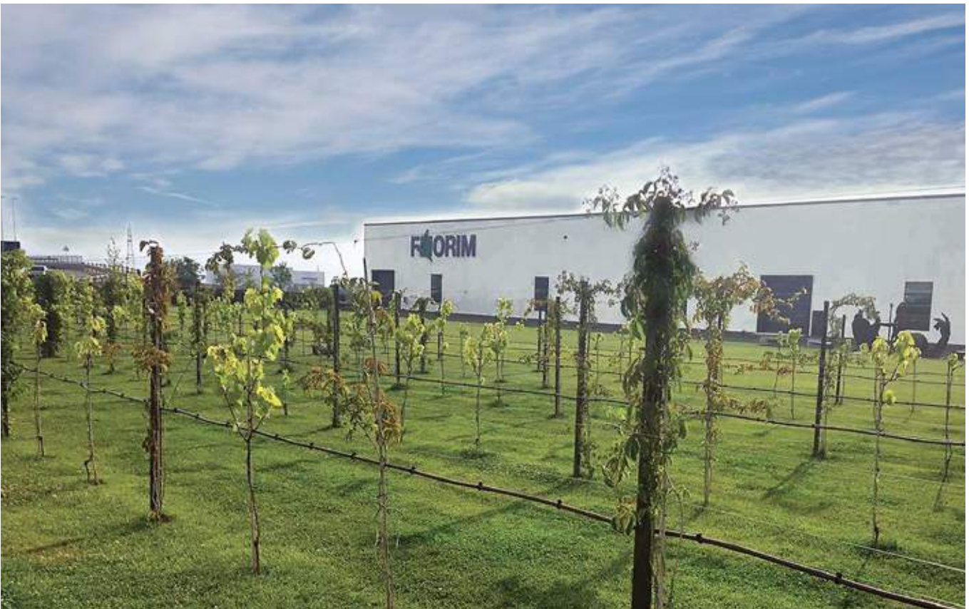
Florim | Industry 4.0 Factory - Plant 2 (Fiorano Modenese - Modena, Italy)
