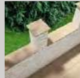
PARAPETS AND FLOWER BEDS trim tiles
